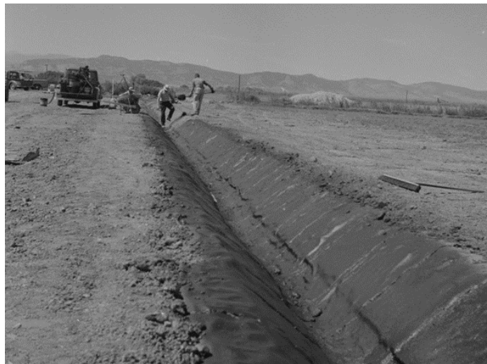
Burlap-asphalt ditch lining being installed at CSU's Research Farm, Summer, 1959. CSU Archives. Photo by Ivan Wood.
